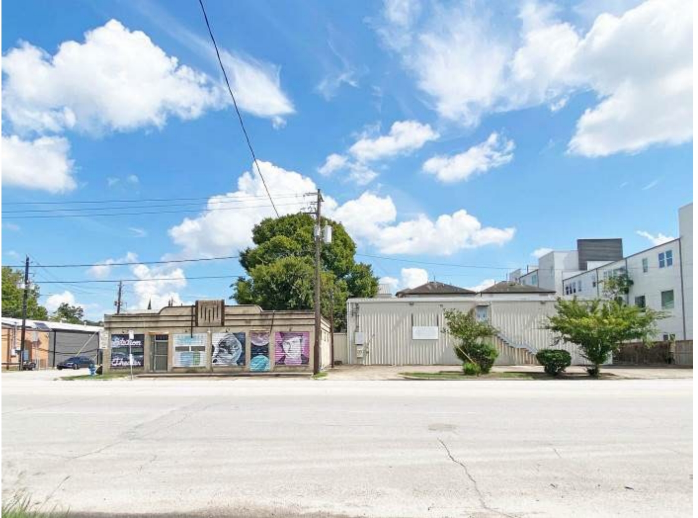
Figure 12: Photograph of Knapp Chevrolet Building Circa 2021 with Previously Connected 1990's Addition (1224 Houston Avenue) Prior to Rehabilitation.
