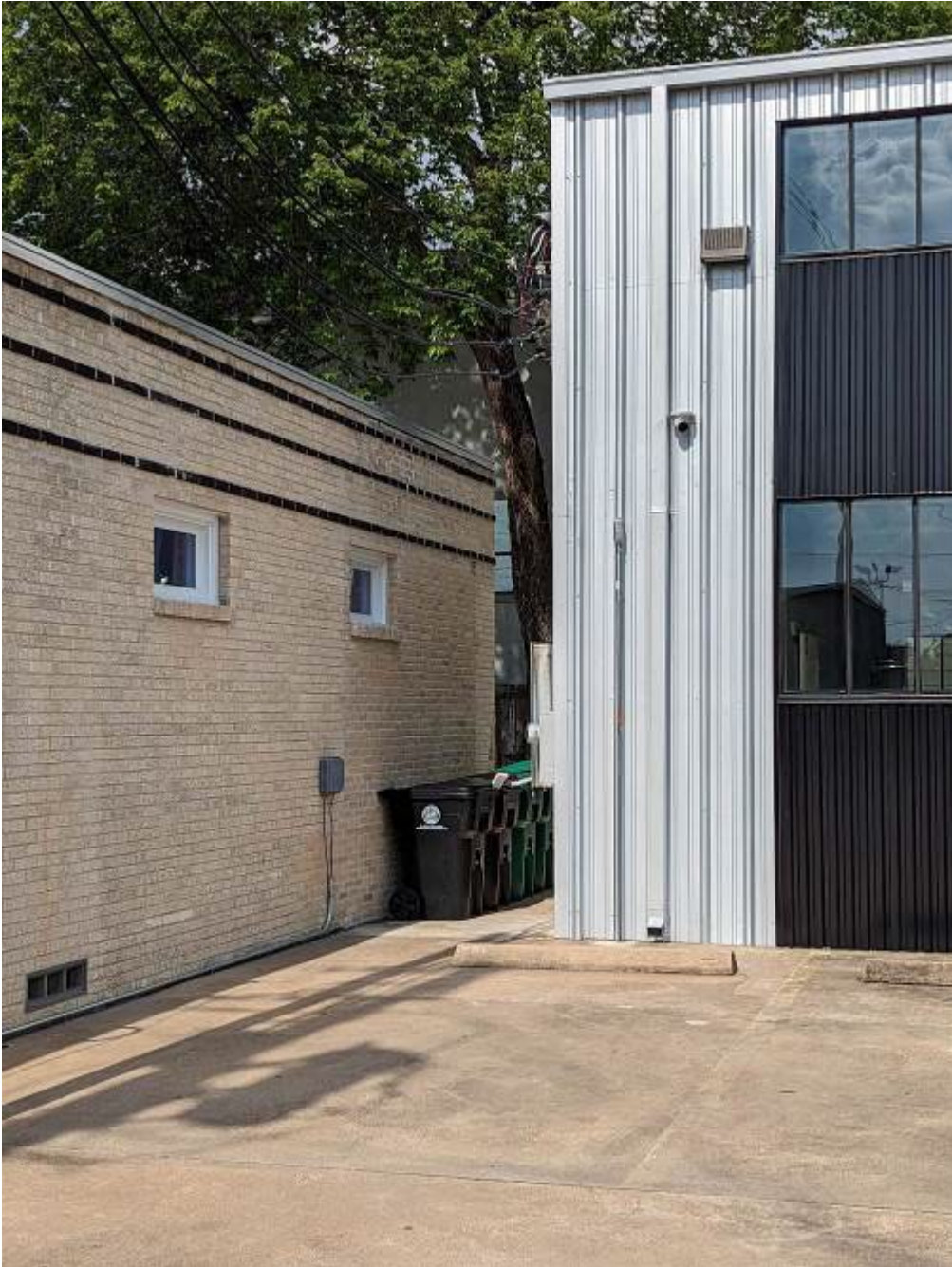
Photo 8: South Façade View Looking East at location of previous connection to adjacent metal building. 8 June 2023.
