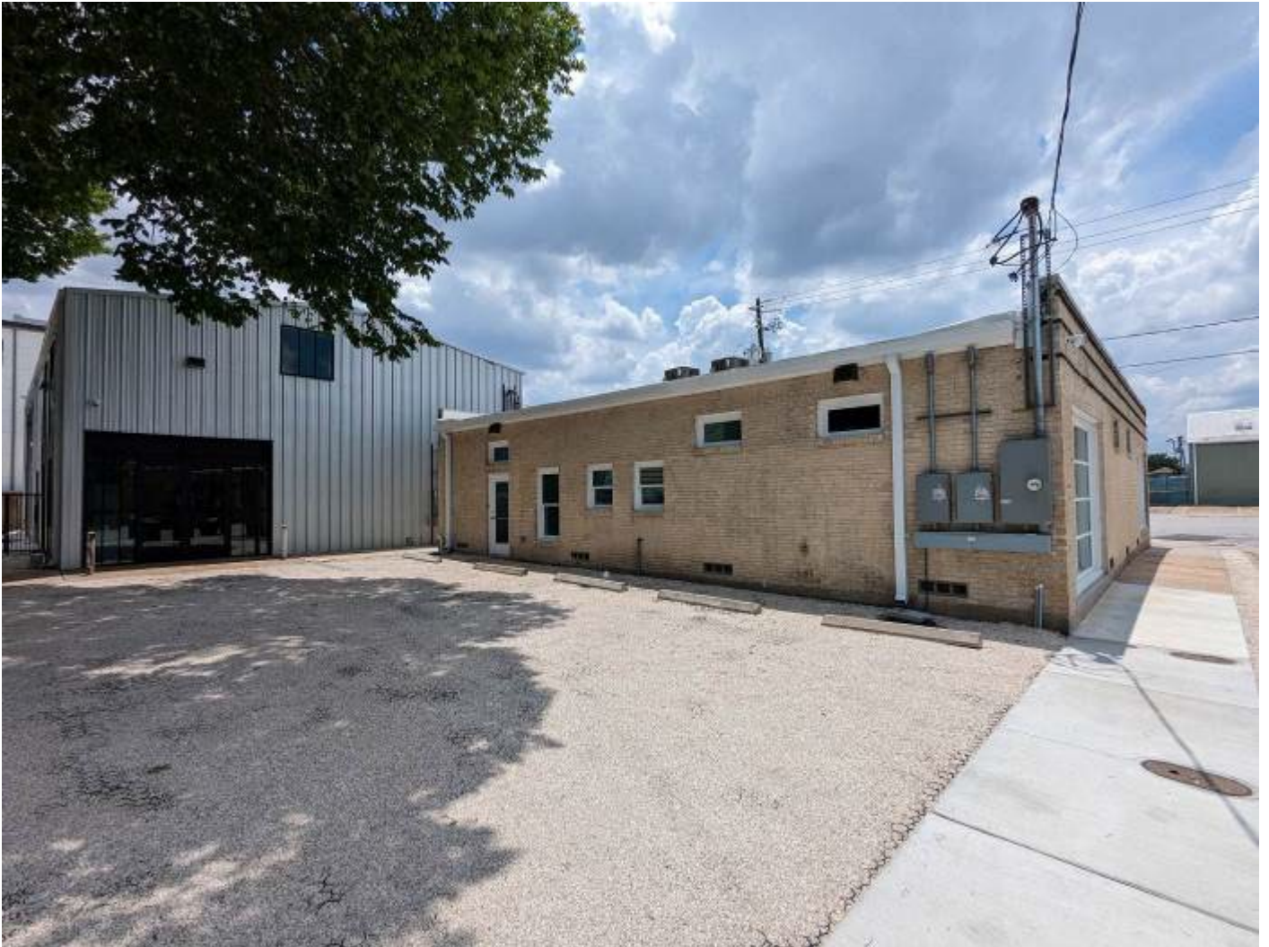
Photo 5: East (Rear) Façade with adjacent building 1224 Houston Avenue. 11 June 2023
